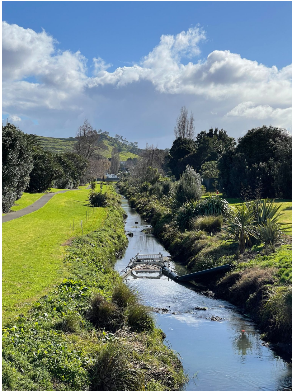
Litter trap collecting plastics and other inorganic matter to prevent the pollution of the Te Ara-rata Stream.
