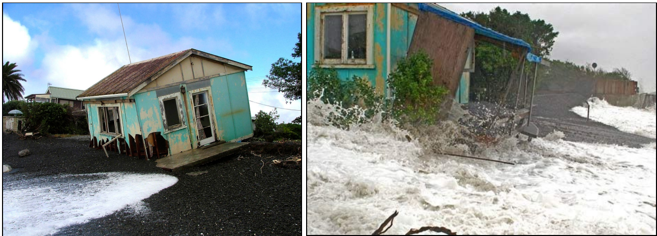
The first home in Haumoana to be destroyed by the sea - photos by Alan Blacklock and Te Ara
